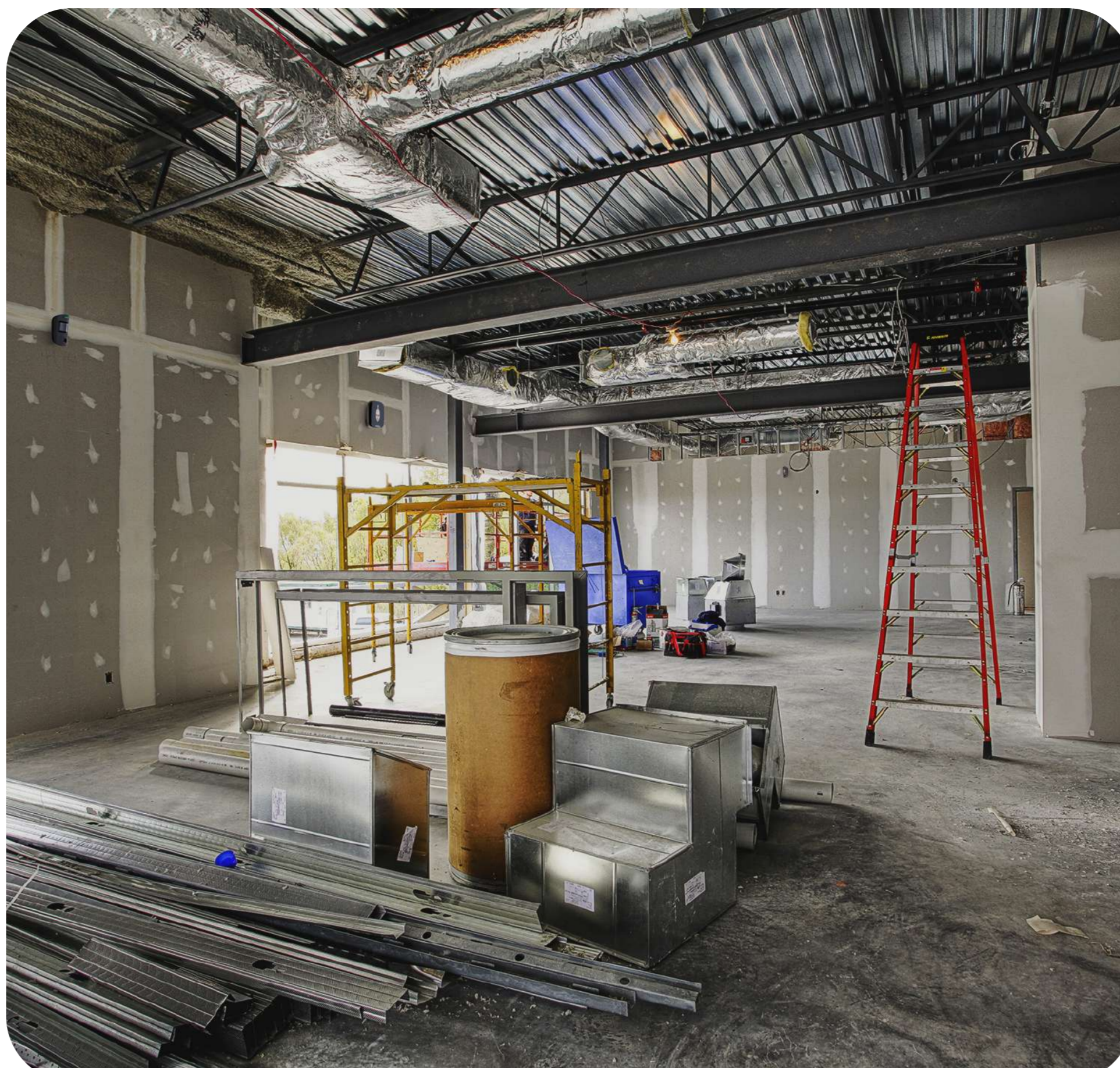
Active or frozen construction with high-cost materials and equipment inside
